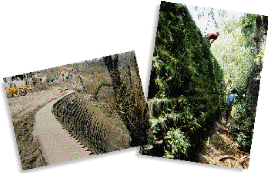
Vegetated Earth Retention Structure Milton, Ontario Canada
