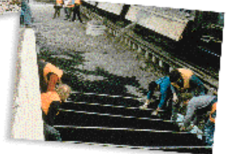
Track Sub-ballast Load Support Over Peat Bogs Eastern Region, England
