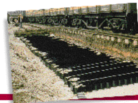
Track Sub-ballast Load Support Over Peat Bogs Eastern Region, England
