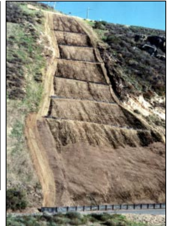
Slope immediately after infill of cells.
