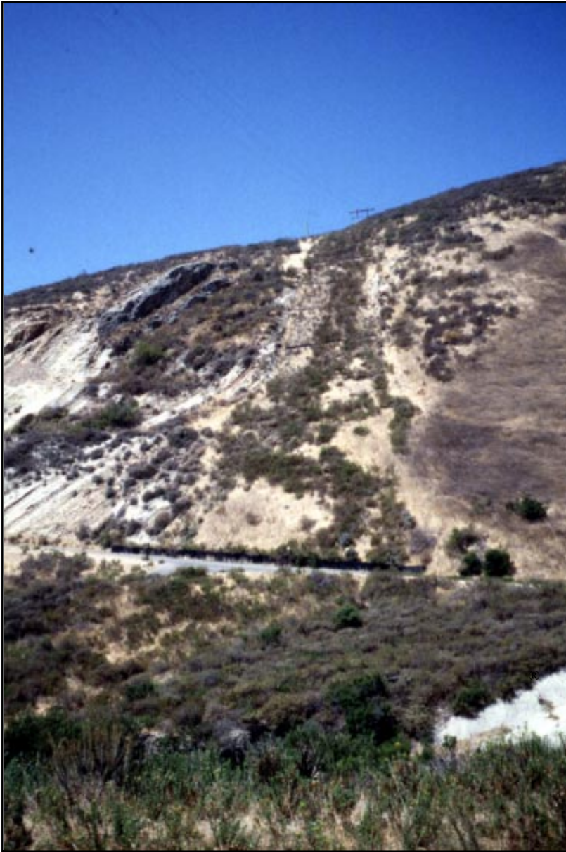
After repair, vegetation beginning.
