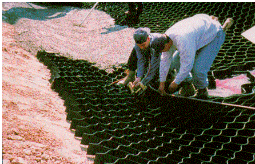
Connecting adjoining Geoweb sections with a pneumatic stapler
