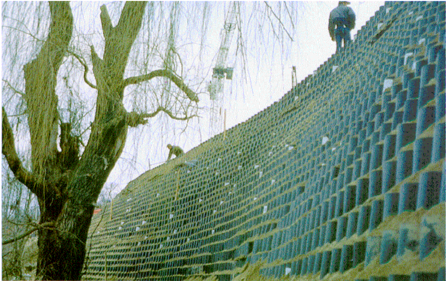
The Geoweb system's steep embankment conforms to a contoured landscape and space constraints, allowing the preservation of several willow trees.
