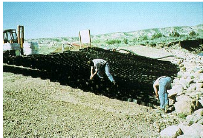
After discarding other alternatives, park officials decided to install a cellular-confinement system. It took just one afternoon for a three-man crew to install the 75 geocell sections needed for this project.
