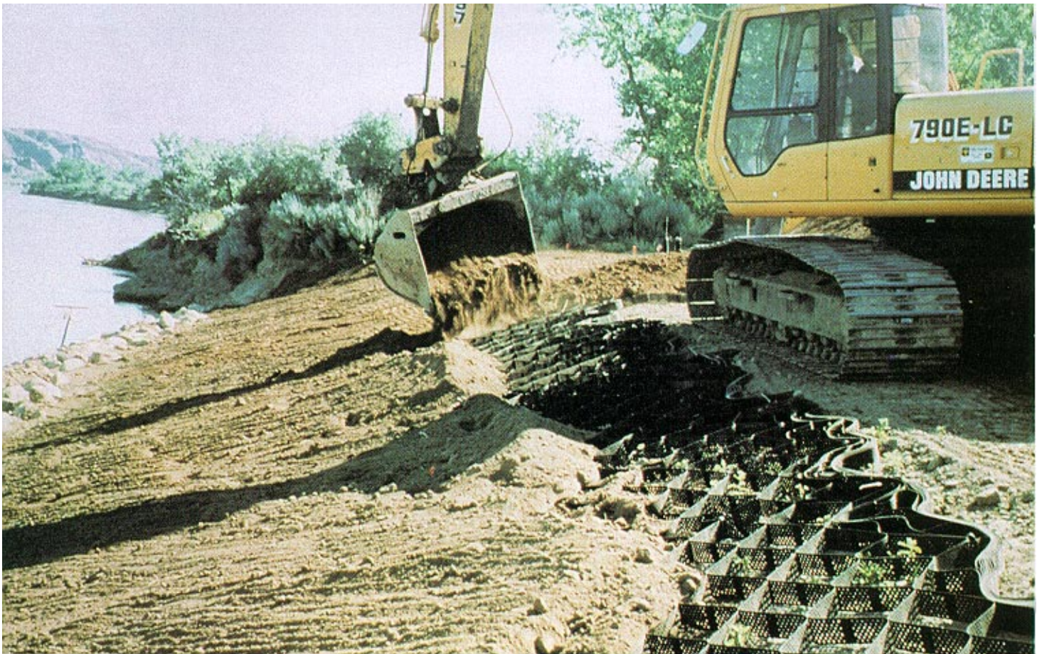
A cellular-confinement system provides structural support to the soil veneer and ensures that a uniform soil thickness is established and maintained on the slope face.
